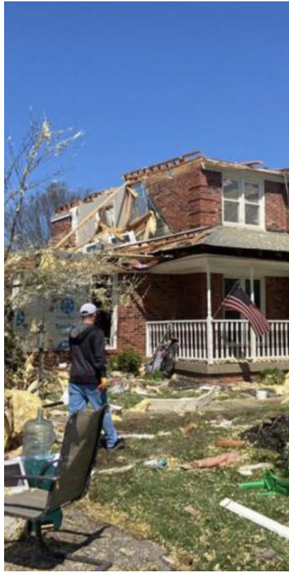
Above: A home in Louisville, Kentucky, destroyed by a tornado. Photo/WDRB.com.
